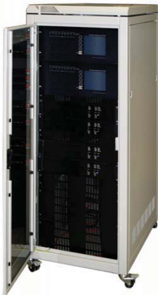
rack mounted panels
